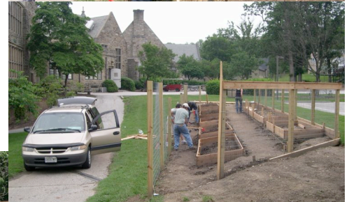
Construction during May & June ↑
